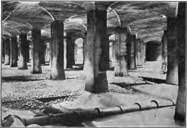
FIG. 43a.—Filtration beds showing connection with water mains.
